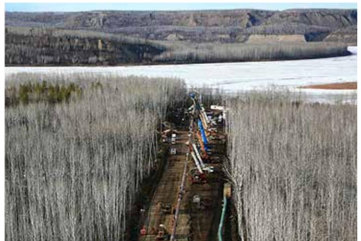
*Horizontal Directional Drilling (HDD) is a trenchless method of installing pipe in a number of geotechnical conditions such as watercrossings. Both banks and the riverbed were not touched during construction.*
